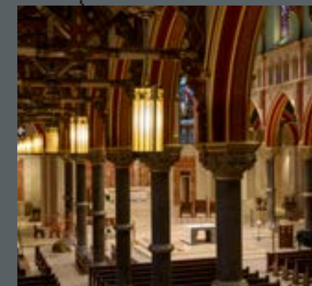
New lanterns with LED illuminators
